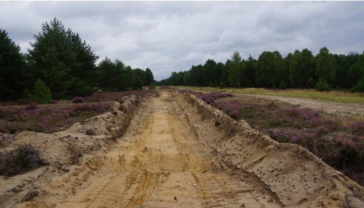
Figure 11: Firebreak created by remote-controlled caterpillar. For further explanations, see text.
